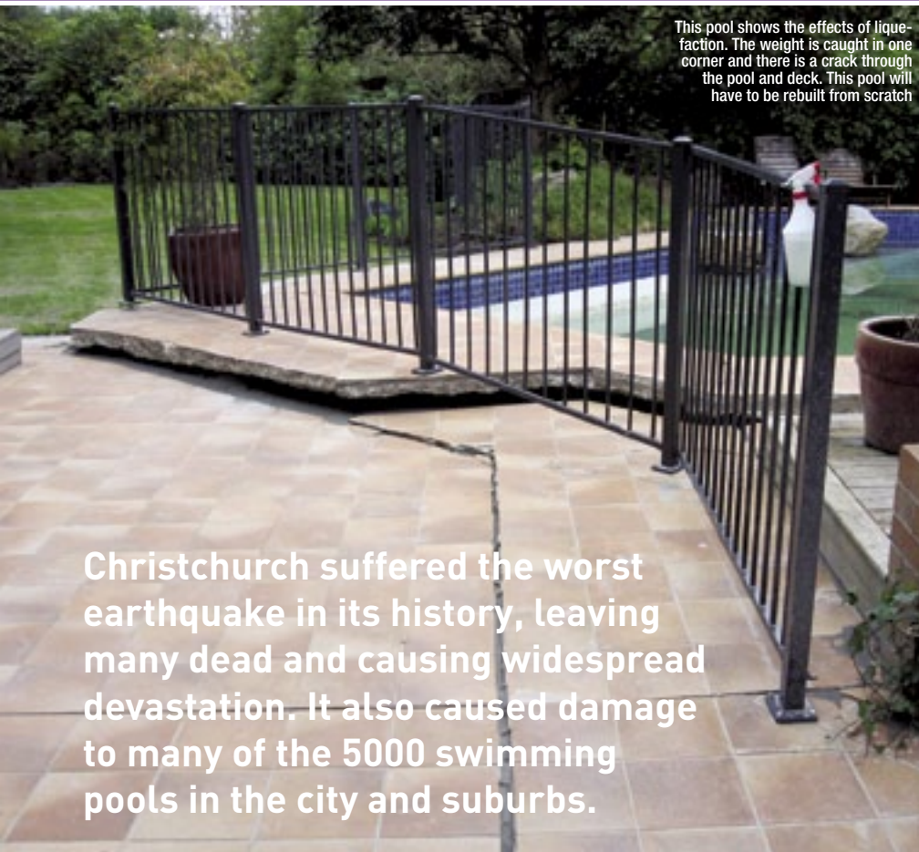
Some pools with only a crack in the corner or a hairline crack are repairable.
