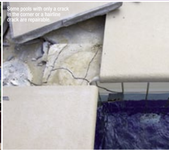
This pool shows the effects of liquefaction. The weight is caught in one corner and there is a crack through the pool and deck. This pool will have to be rebuilt from scratch
