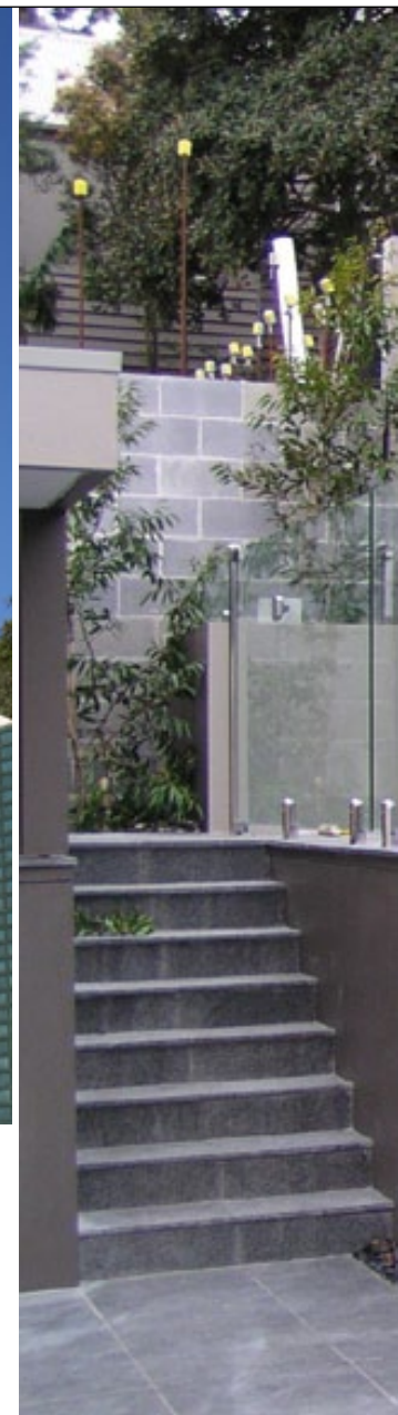
RIGHT: On this particular job, fencing is installed where there would otherwise be access, but is not required in the central section with the glass pool wall, because it is already more than 1.2m high. De Fence
