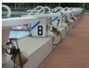
Dive blocks have individual speakers and touch buttons as back up for time keepers
