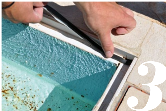
Adhere the anti-vibration tape to the ledge
