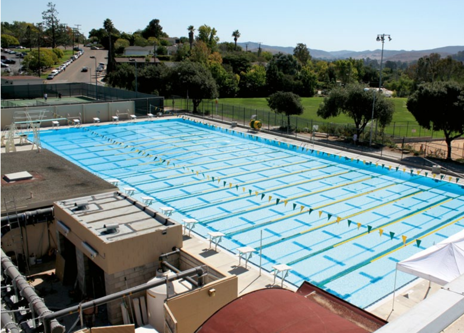
Myrtha Pools' California Polytechnic State University project in San Luis Obispo, California
