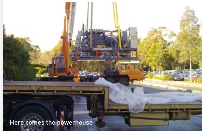
The six-cylinder MAN engine produces 775,320kW of electricity per year which has reduced energy costs dramatically
